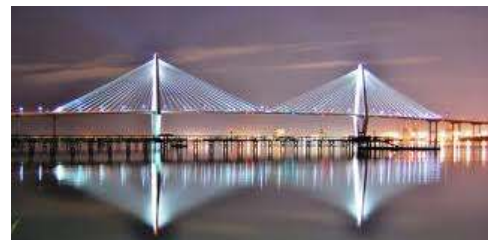
New Cooper River Bridge
