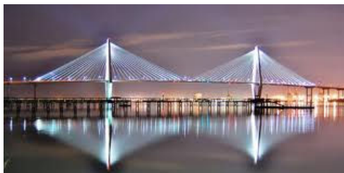
New Cooper River Bridge
